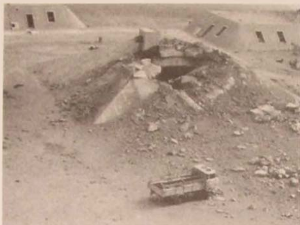
Iraqi bunker destroyed by a laser-guided bomb
